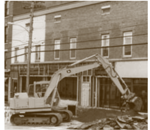
Work begins on expansion of the main NSB office in 1973.
