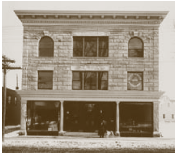
The Barre branch, as the building looked when built in 1904. Pictured are Angelo Scampini and his dog.
