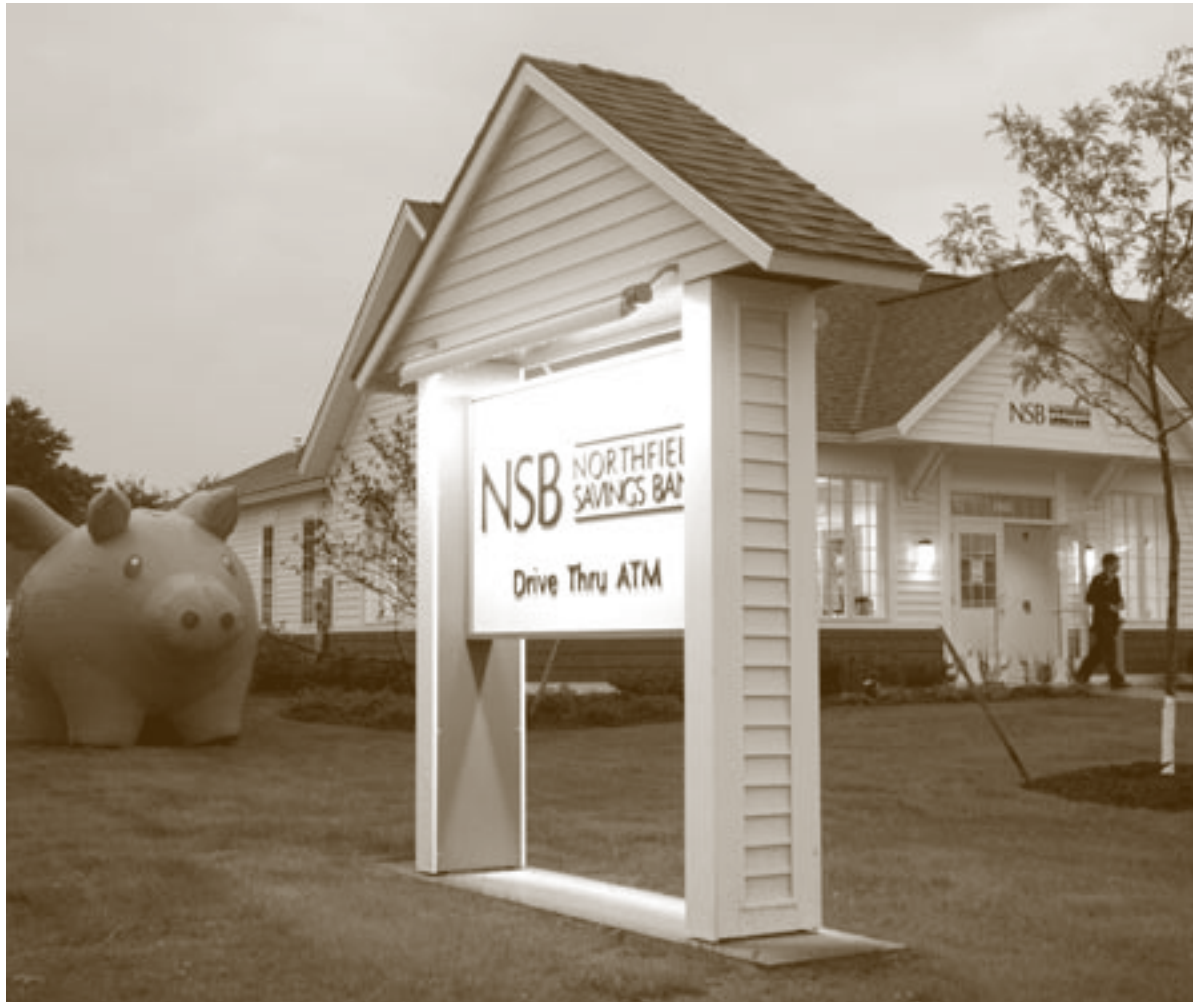
This NSB office located on Williston Road in South Burlington is the fifth branch built during expansion into Chittenden County.
